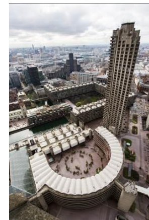
9. Aerial view of the Barbican Centre CREDIT Sidd Khajuria
